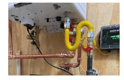
Please note: The Flow-Tech MAX Anti-Scale System relies on a return path to ground to work effectively. The initial grounding source is obtained through a properly grounded electrical outlet. The return path is most typically obtained through a conductive metal path to a grounded water heater. In the event that neither of these options are achievable, ground can be reached via a properly grounded gas line or properly grounded plumbing system.
